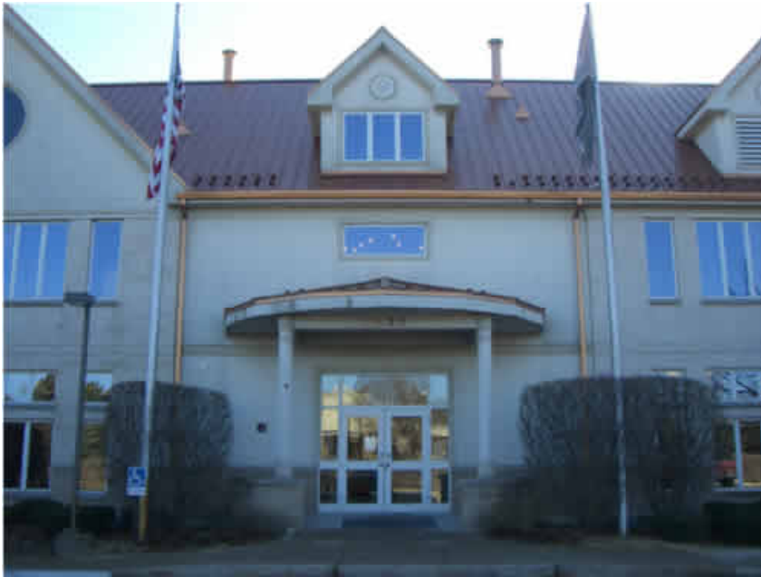
Moisture readings checked ok
