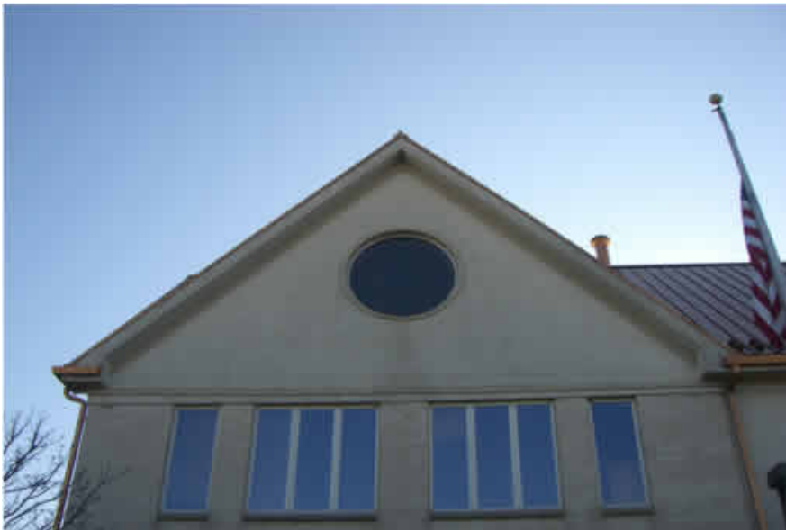
Moisture readings checked ok (typical)
